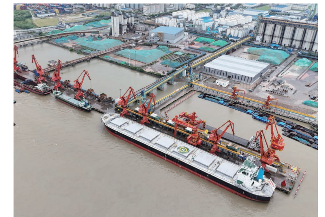
Taizhou Yonggan Dock Renovation Project
