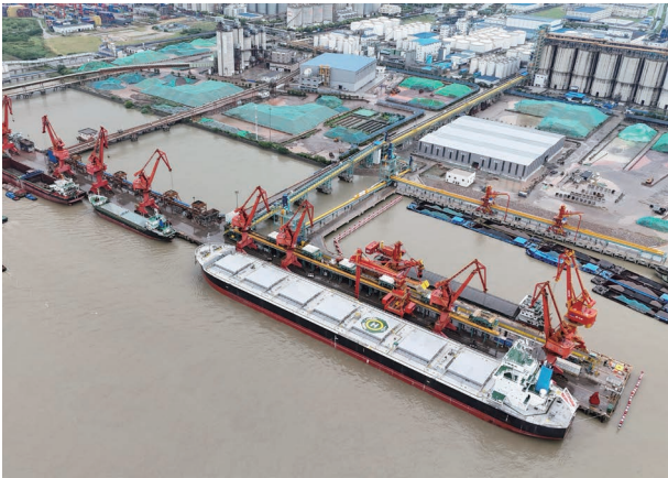
Taizhou Yongan Dock Renovation Project
